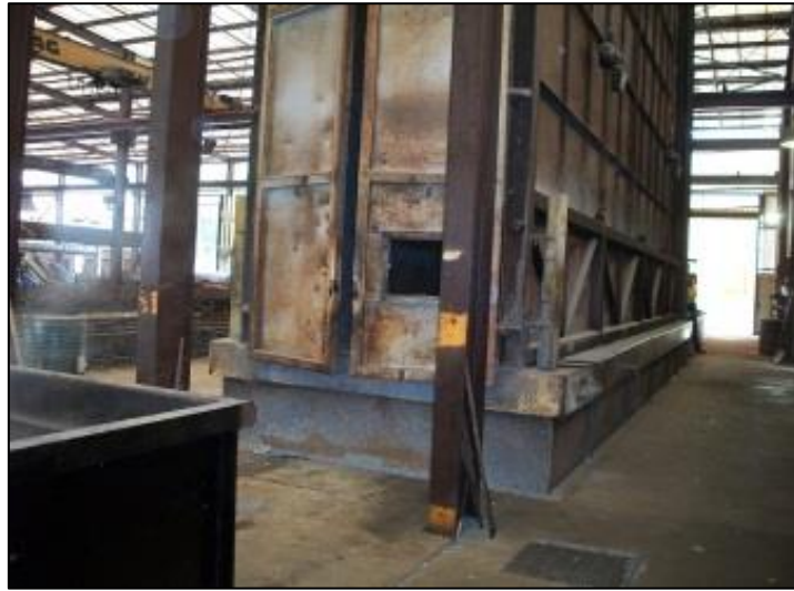
Figure 1-5: Plant 1 galvanizing bath with enclosed kettle hood
